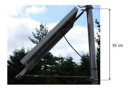
When positioning the solar panel it should always face true south if you are in the northern hemisphere, or true north if you are in the southern hemisphere. True north is not the same as magnetic north. If you are using a compass to orient your panels, you need to correct for the difference, which varies with location. Search the web for "magnetic declination" to find the correction for your location.
